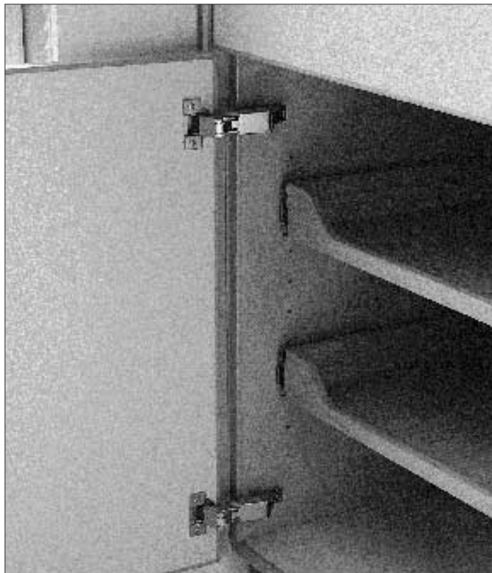
Figure 2. Cup hinges are available in a wide variety of configurations for different cabinet locations and door reveals. The author uses a 165-degree hinge for base cabinets, which opens the door out of the way of the sliding trays.
