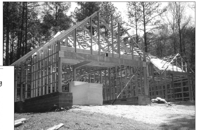
Figure 1. This pre-engineered frame, made by Advanced Framing Systems, uses hat-shaped horizontal channels to reduce thermal bridging through the wall.
