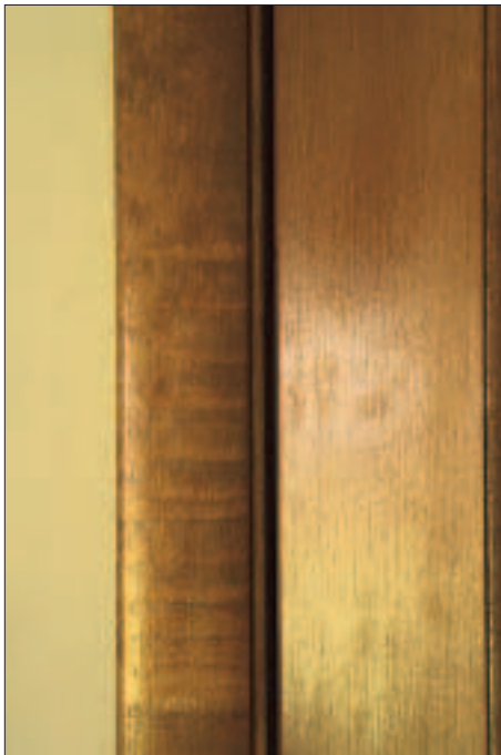
Figure 3. According to AWI standards, economy-grade trim, like this stock clamshell, can show as few as 15 knife cuts per inch. The material shown here is much coarser and should have been rejected.
