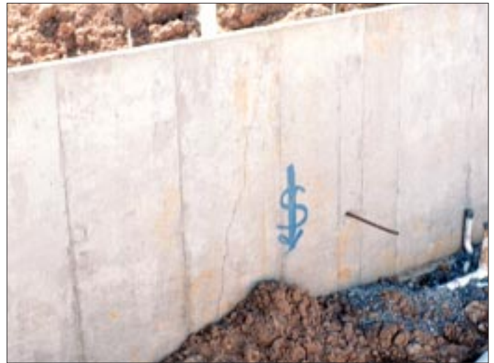
Figure 2. Backfilling an unbraced wall can result in bows (left) and cracks (right). Fixing these problems requires excavation, pushing out the wall, and installing new waterproofing — at a cost much greater than doing the job right the first time.
