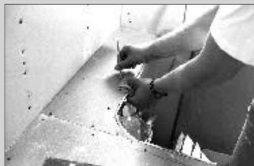
(B) To ensure an accurate layout, he draws a line parallel to the sink-metal edge, using a sample tile for exact measurement.
