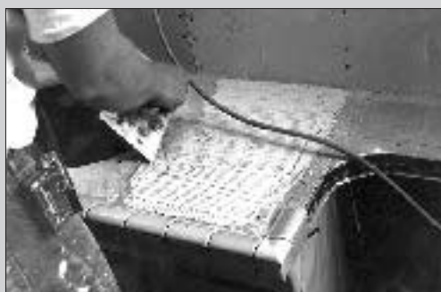
(E) With the edge tiles in place, the author spreads the thinset with a \frac{1}{8} -inch square-toothed trowel.
