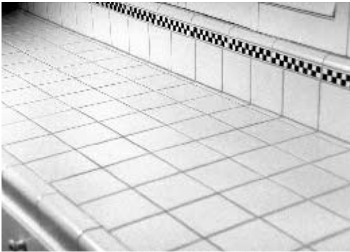
Figure 2. Poor tile layout. Instead of leaving a narrow strip of tile along the backsplash, the tilesetter should have used one less full tile and set two "half" tiles at front and back.
