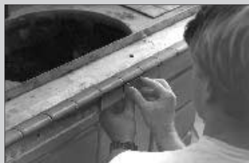
(D) The edge tiles are set first, beginning at the outside corner and working towards each end.
