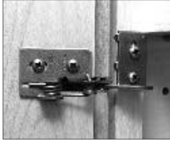
Figure 5. Knife hinges are partially concealed and are adjustable in two dimensions.
