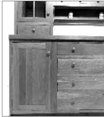
Figure 3. With inset doors, a gap is visible between the doors and drawers and the cabinet frame. Expansion and contraction may cause the fronts to rub against the frame.
