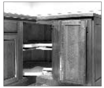
Figure 7. Many corner cabinets now contain a Super Susan, which rides on ball bearings on the cabinet bottom or on an intermediate shelf, eliminating the need for a center post.
