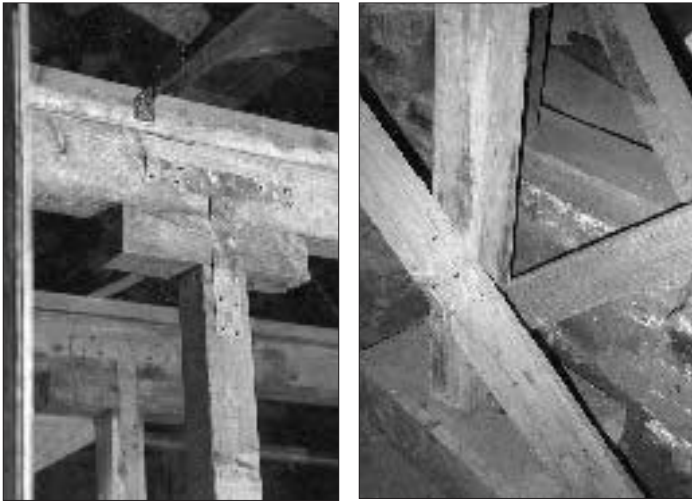
Figure 3. Shoring details. The author uses 4x6 girders and 4x4 posts to support the building before demolishing the old foundation. He snugs the posts into place with wedges cut from 4x4s, nails them in place with duplex nails, then reinforces the whole connection with a metal T (left). At the base, the posts rest on 8x8 blocks that have been sandwiched between 3/4-inch plywood (right). This prevents the wood from splitting as it takes on and loses ground moisture.
