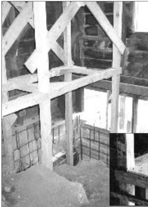
Figure 3. Shoring details. The author uses 4x6 girders and 4x4 posts to support the building before demolishing the old foundation. He snugs the posts into place with wedges cut from 4x4s, nails them in place with duplex nails, then reinforces the whole connection with a metal T (left). At the base, the posts rest on 8x8 blocks that have been sandwiched between 3/4-inch plywood (right). This prevents the wood from splitting as it takes on and loses ground moisture.
