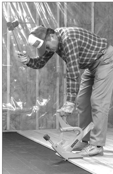
The debate over the suitability of OSB as a subfloor under hardwood strip flooring continues to yield mixed results.
