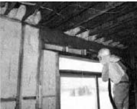
Icynene does a good job of insulating odd-shaped cavities, such as at the band joist (left) and around doors and windows (right).
