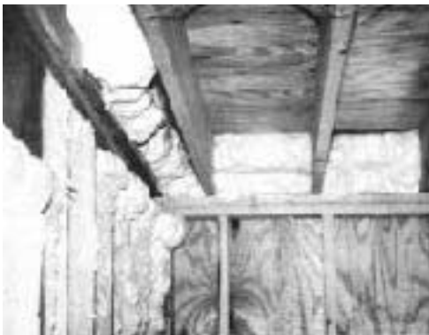
Icynene does a good job of insulating odd-shaped cavities, such as at the band joist (left) and around doors and windows (right).
