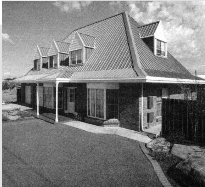
Ag-panels are widely used on house roofs. But because residential roofs are more complicated than the agricultural buildings the roofing was designed for, a builder must use premium metal coatings, factory-finished panels, and watertight details.
