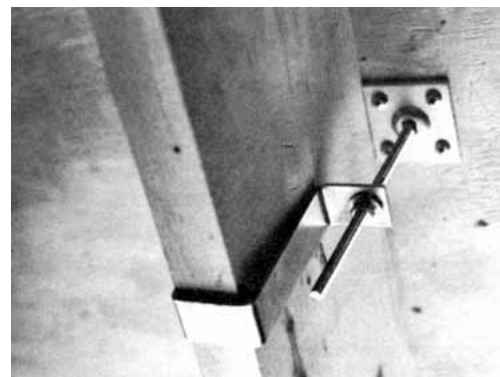
Figure 2. Two ways to fix squeaky floors: The Floor Binder (left) has inclined nail slots, so as you drive the angle-iron sideways, the floor joist and subfloor are drawn together. The Squeakender (right) hooks under the joist, and pulls the subfloor down as the nut is tightened.
