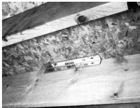
Figure 2. Two ways to fix squeaky floors: The Floor Binder (left) has inclined nail slots, so as you drive the angle-iron sideways, the floor joist and subfloor are drawn together. The Squeakender (right) hooks under the joist, and pulls the subfloor down as the nut is tightened.
