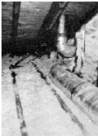
Air Krete, a cementitious foam insulation, is free of the toxins found in many conventional insulation products.
