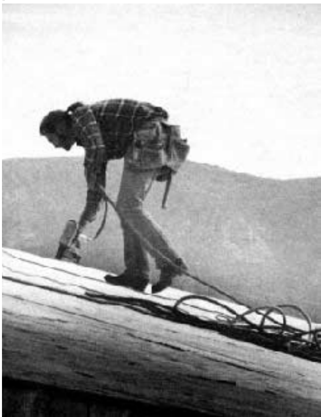
Davis warns his framers to release the nail-gun trigger between shots. In the past, one framer shattered a finger by "bounce nailing." Another had to have a 16d nail surgically removed from the ball of his ankle.
