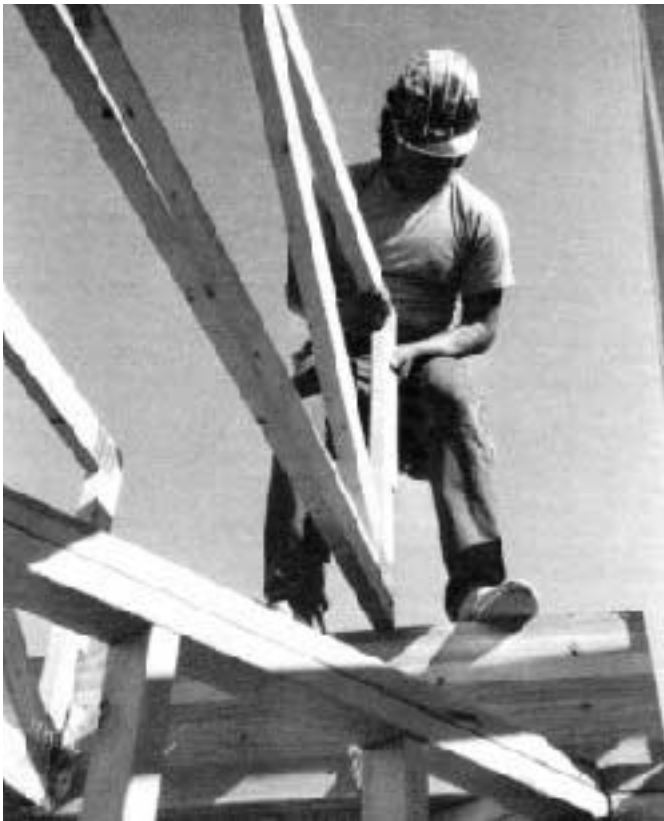
On large, multi-story commercial sites, Davis's framers wear hard hats. He requires boots and safety glasses on all his sites to minimize small injuries like nail punctures and sawdust in the eyes.
