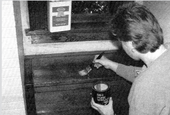
Shellac works well as a sealer under pigmented stain or as a primary finish. Its main advantage as a finish is the ease with which you can repair drips or scratches.
