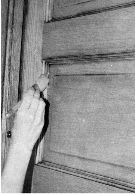
For a panel door, start with the ribbon mold, using a 1 1/2-inch diagonal "sash tool." Then do the panels, the center stiles, the cross rails, and the two end stiles.
