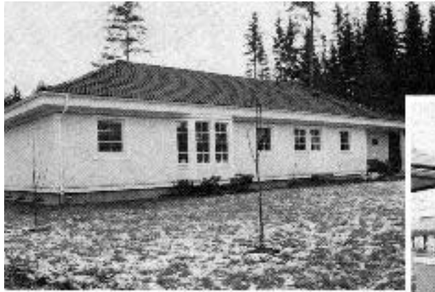
The typical factory-built house in Sweden (left) has board-and-batten siding and a tile roof. With Japanese manufactured homes (below), customers use computers to choose among a host of custom features and finishes, many mimicking U.S. designs.
