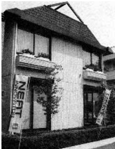
Figure 4. This Misawa home is built with PALC panels, one of Japan's newest building materials. PALC, a lightweight concrete, is reinforced with steel mesh and stamped with different colors and patterns.
