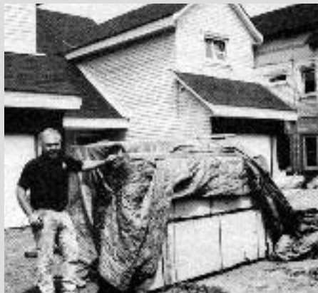
Builder Ron Bardenhausen erected panelized townhouses that were shipped from Sweden. Storing all materials on site caused some frustrations.
