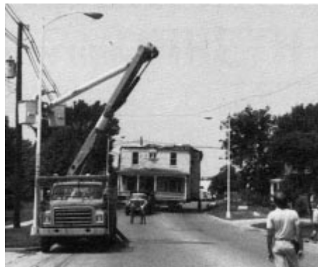
Figure 1. This house required tree trimmers to cut back branches because it was too wide for the road. Fifty feet ahead of the house, phone company workers drop a low hanging line.
