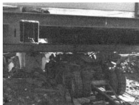
Figure 4. A cable from the truck loops around the pulley on the front dolly.
