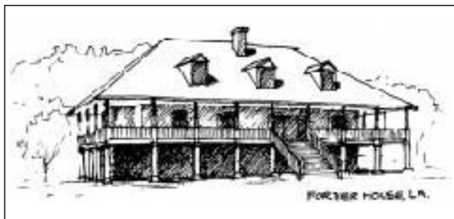
Figure 2. The Fortier House at Homeplace Plantation in St. Charles Parish, La., is a classic example of how hip roofs can cap off porches on French Colonial homes.
