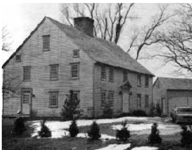
The Park Homestead, fully restored. The restoration used antique glass in all the windows, and blacksmith-made nails were used in all visible woodwork.
