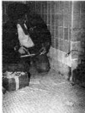
Figure 2. Unglazed porcelain tile was used on the floor in this gym shower room, but the walls take a glazed tile. Porcelain tile is a low-absorbency, vitreous tile.
