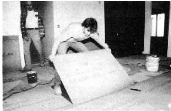
Figure 5. Cement backer board must be laminated to the subfloor beneath it. Use an approved water proof adhesive and apply it to fully cover the plywood surface.
