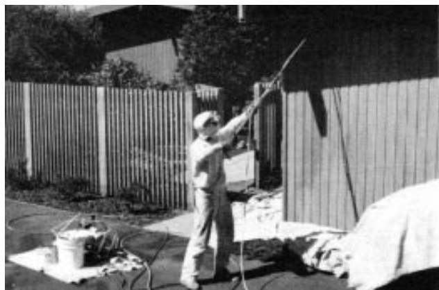
Figure 2. With rough-sawn textures and grooved plywood siding, brush and roll the first coat for good penetration and even distribution. Subsequent coats can be sprayed as shown above.
