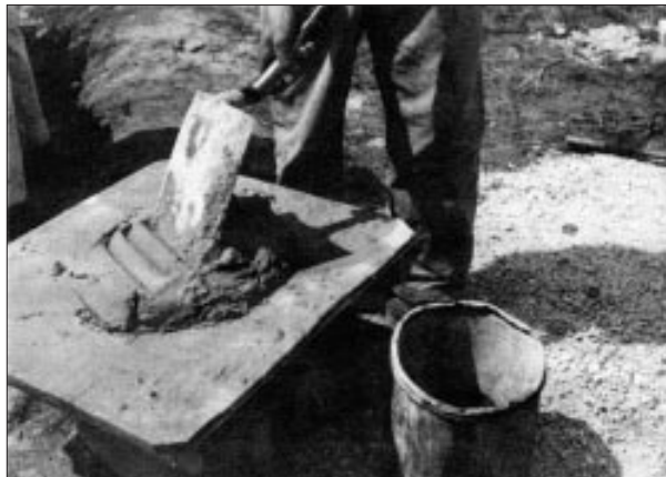
When mortar stiffens due to evaporation, you can "retemper" it by adding water and mixing thoroughly. If it stiffens from hydration - especially if it has been sitting for more than 2 1/2 hours - discard it.
