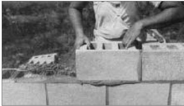
Mortar should be workable enough to spread easily, and plastic enough to extrude from joints without dropping.
