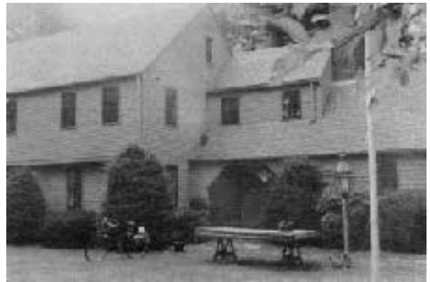
Figure 3. The shrubbery looks nice, but slows down the drying at the bottoms of the outside walls.
