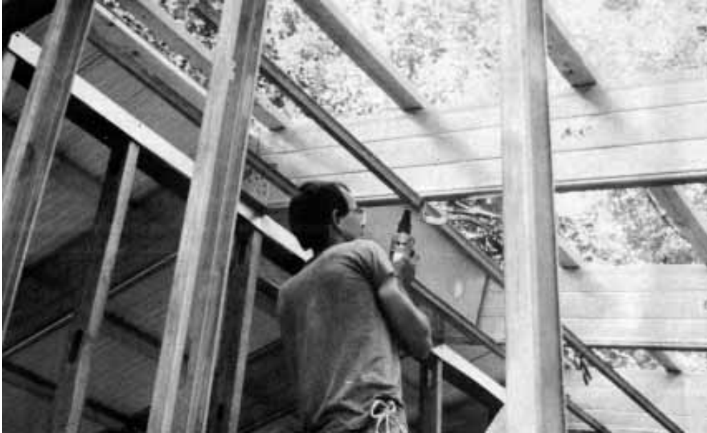
The author installs steel framing members to avoid using wood or wood products, which can make some people sick due to outgassing.
