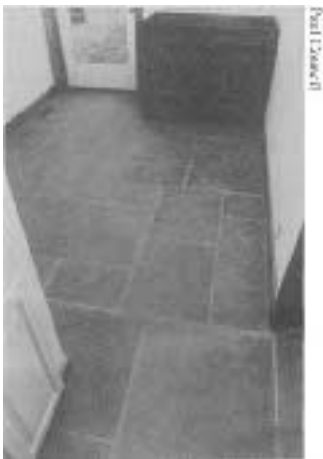
For an appealing pattern, mix large and small stones and avoid long, continuous joints.
