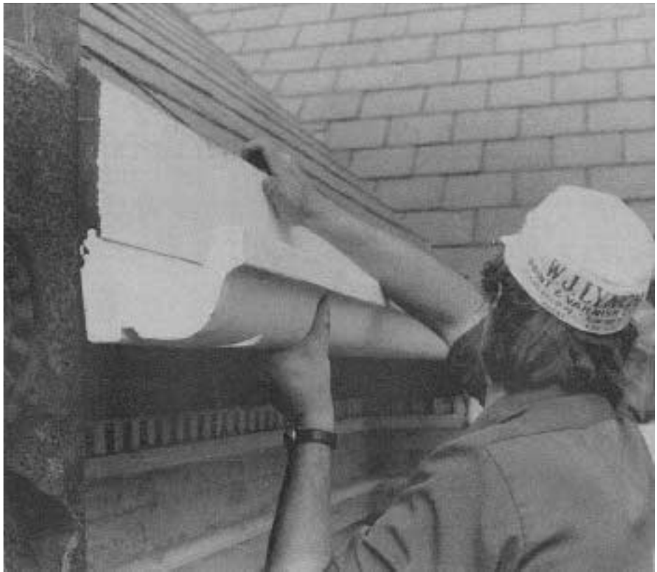
Figure B. Installing a new gutter section.
