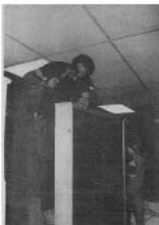
▶ Max Headroom As fresh panels come rolling off the assembly line, editor Steve Bliss trims them out in place.
