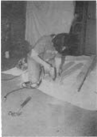
◀ Cover-Up Drop cloths kept sawdust out of the computer disk drives, but the carpeting could have used a bit more coverage. Here managing editor Kate O'Brien pre-drills the ends of plates to accept long wood screws.
