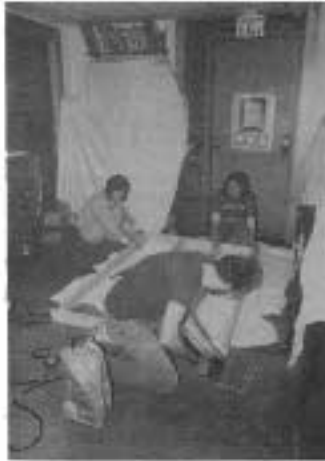
◀ Cover-Up Drop cloths kept sawdust out of the computer disk drives, but the carpeting could have used a bit more coverage. Here managing editor Kate O'Brien pre-drills the ends of plates to accept long wood screws.
