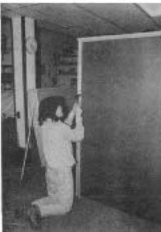
▶ On Schedule At day's end, all eight sections are in place, and the carpet vacuumed. By designing around the materials, there was minimal cutting and virtually no waste.
