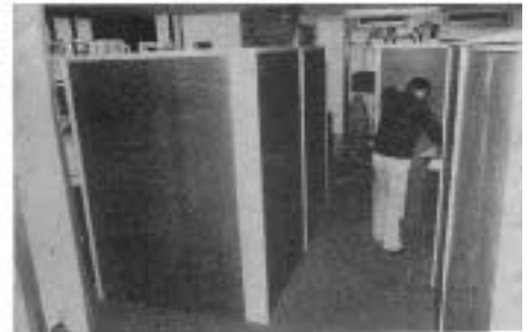
▶ On Schedule At day's end, all eight sections are in place, and the carpet vacuumed. By designing around the materials, there was minimal cutting and virtually no waste.
