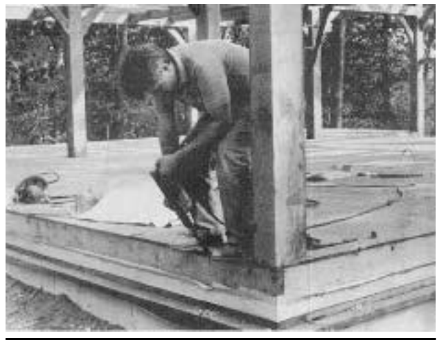
The lower sill, shown in the detail below, is extended out to support the wall panels. The upper sill and deck can be made of timbers, or can be conventionally framed, as in the photo above, where the box sill is being drilled for wiring.
